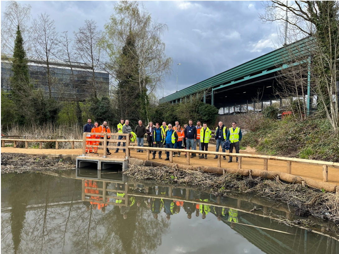
The Site team with Directors; Joe Paine, Alistair Maidman, Sue Marshall and representatives from Hart district council on a tour of the works before being officially reopened to the public.
